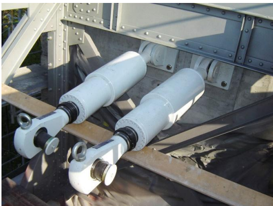
Figure 40 Example of a shock absorber
