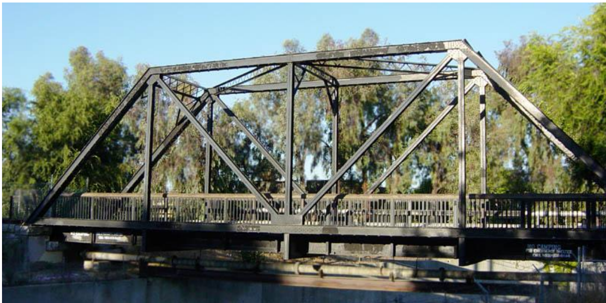
Figure 24 Example of a truss
