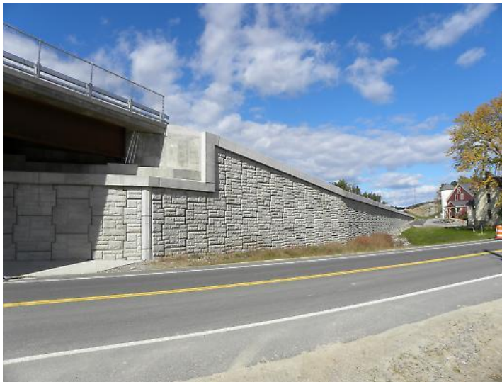
Figure 9 Example of a retaining wall
