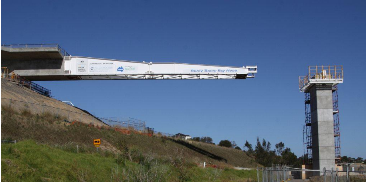
Figure 58 Example of a Launching nose
