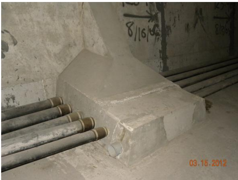
Figure 49 Example of a deviator
