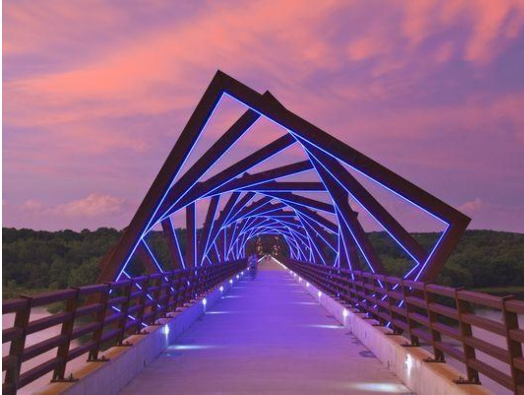
Figure 56 Example of lighting on a bridge
