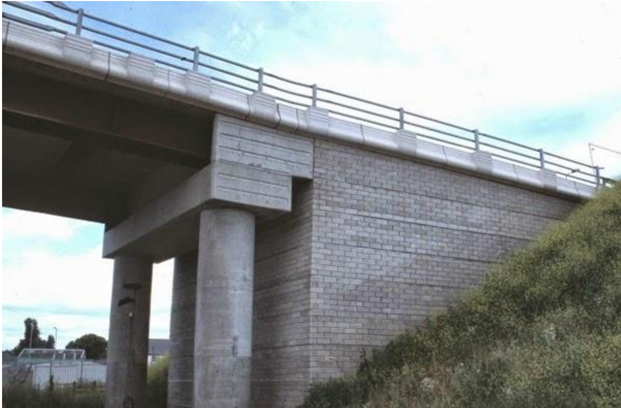
Figure 6 Example of an abutment
