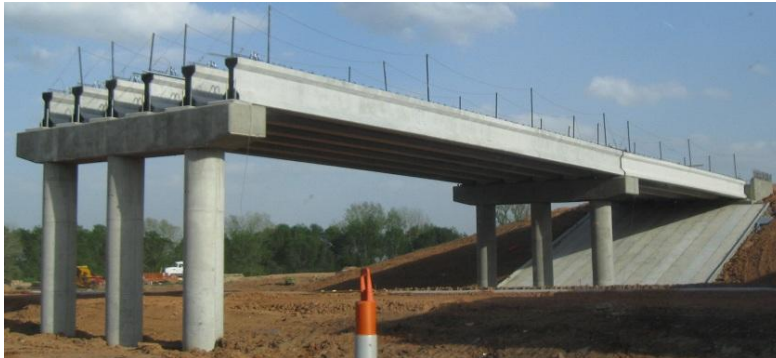
Figure 7 Example of a pier
