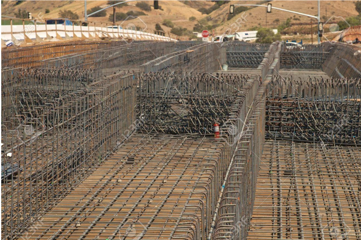
Figure 42 Example of a rebar array
