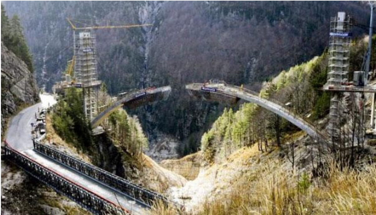
Figure 60 Example of a staying mast
