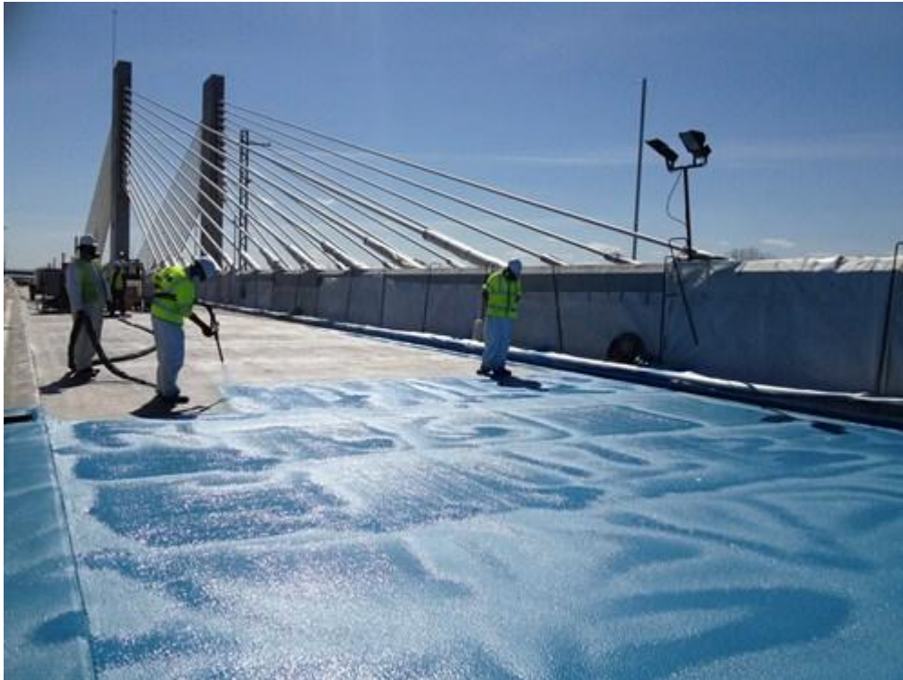
Figure 32 Example of a waterproofing membrane
