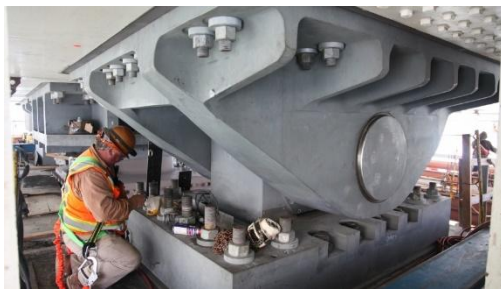
Figure 35 Example of a bearing
